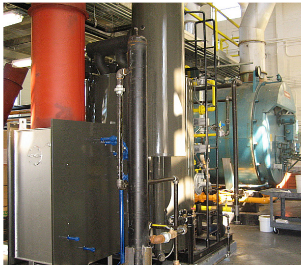
Ethicon Cornelia, GA Boiler Upgrade
