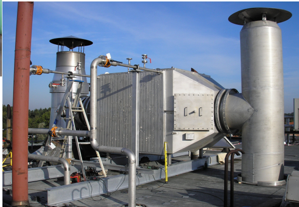
Janssen Beerse, Belgium Stack Gas Recuperation
