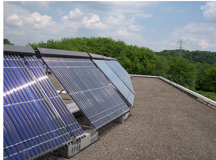
McNeil Consumer Ft. Washington, PA 124 kW Thermal System for Boiler Pre-heat
