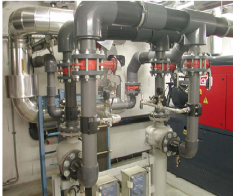
DePuy - St. Priest, France Geothermal Heating / Cooling System
