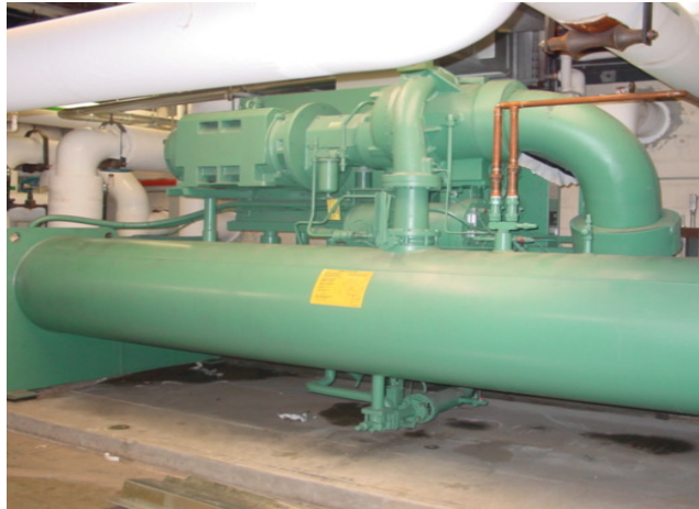
Ethicon Somerville, NJ Upgraded Chiller with VFD
