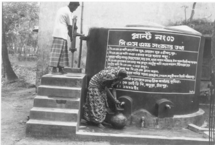
Figure 7. Ponds Sand Filter
