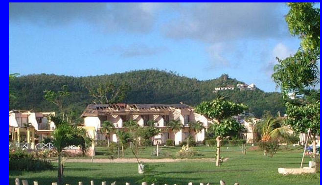
Damage by Ivan (Grenada)
