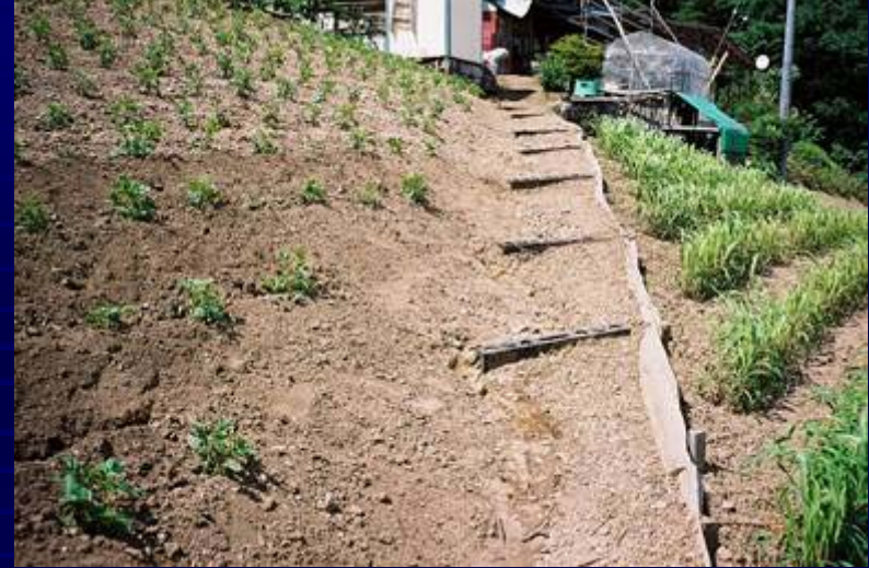
Installation of the materials which prevents soil erosion.
